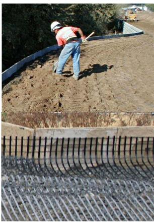
Now carefully backfill over the grid, to the top of wall panel, keeping the geo-grid tight and free of wrinkles., A minimum of 2 foot of select material is to be maintained at the wall face. Compact as previously described beginning over the tail of the counterfort to the panel back and then toward the back end of the geo-grid Insure that the geogrid remains in contact with the panel back after compaction
