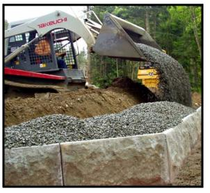
For rows that will contain soil reinforcement the grid is placed after the first lift of fill is compacted so that geo grid is located at about the mid-point of the wall panel.
