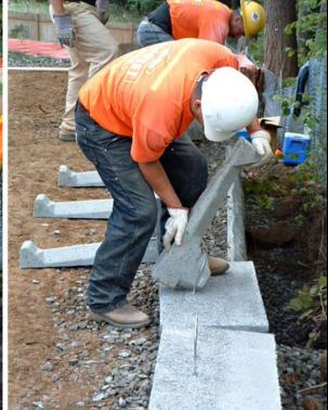
Use wedges between the counterfort head and the panel back to remove play and make the module rigid.
