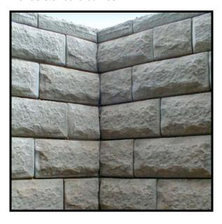
Corners: LOCK+LOAD does not need to be built "on bond" but if it is required, for aesthetic reasons, the panels will need to be trimmed for inside corners. The need to trim panels is due to the wall batter. On inside corners the length of subsequent rows grows by 40 mm or 1 9/16". Using a diamond blade cut off saw mark cuts on panel back according to the attached detail and trim to lengths required to maintain the split bond.
