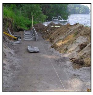
fort until panel is vertical. Place level on top of panel and level horizontally in the same manner. Check top elevation of both panels on each end of wall segment being constructed with laser level to ensure run will be level.
