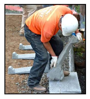
Each **LOCK+LOAD** module consists of two pieces, a panel and counterfort that are easily assembled at the project site; as shown in the picture above.
