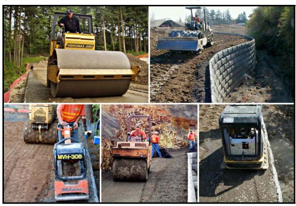
Even better compaction equipment are large the facings attachment to the soil mass. reversible diesel plate compactors with operating weights of 900 to 1100 lbs. [Examples: Wacker models (BPU-3345) or Multi Quip (MVH-200DA) or equivalent]. Roller compactors can safely be used to within 16" of the wall face. All compaction activity always begins with compacting over the tail of the counterfort first "locking" it into place.
