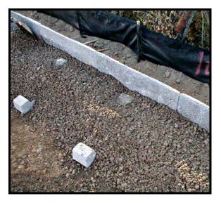
Once select fill material is placed over the counterforts the specified backfill can be placed, leveled and compacted in ~8" lifts within the reinforced soil zone using heavy equipment. Take care not to displace the wall alignment or damage soil reinforcement.
